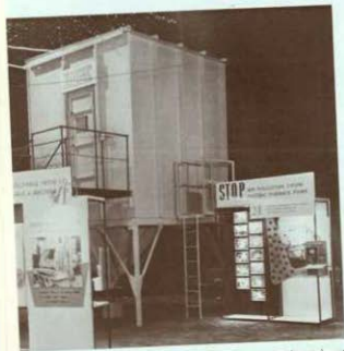
The Dustube Collector which ventilates the Super Tumblers.
