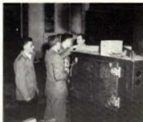
In the Steel Shop, the visitors pause to have a look at a Wheelabrator in the process of construction. With his back to the camera is George McNelle, while Fred Baldauf is at extreme right.
